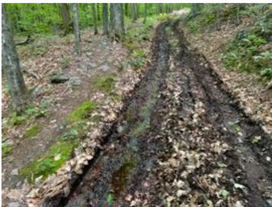
Multiple sections of the ROW are wet and drain through tire ruts.
